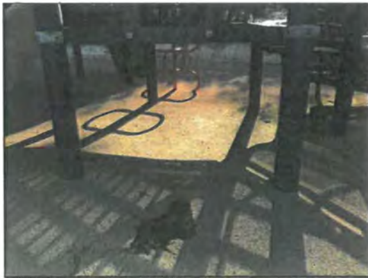
21. Sloped P.I.P. to drain towards center
