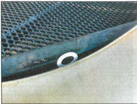
9. Entanglement at small curved slide entry
