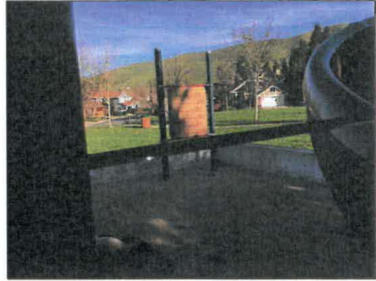
14. Post within slide clearance zone
