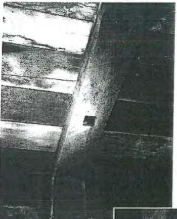
Detail of mortise & tenon construction at wall interior framing (left), 2001
